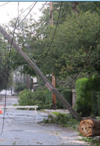
Power lines knocked down by winds from Tropical Storm Irene in 2011, Narragansett.
