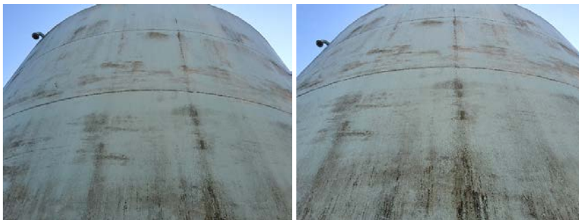
Middle West Wall Section- Photo of welds
