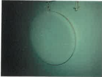
Interior Manway #2 Photos
