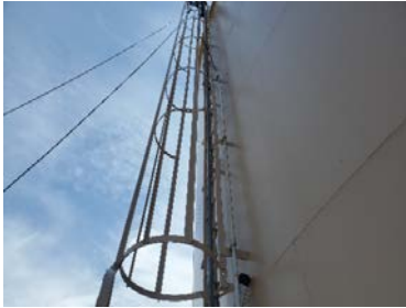
Exterior Ladder Photos
