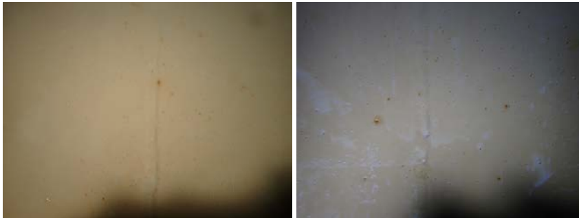
Middle West Wall Section- Photo of welds
