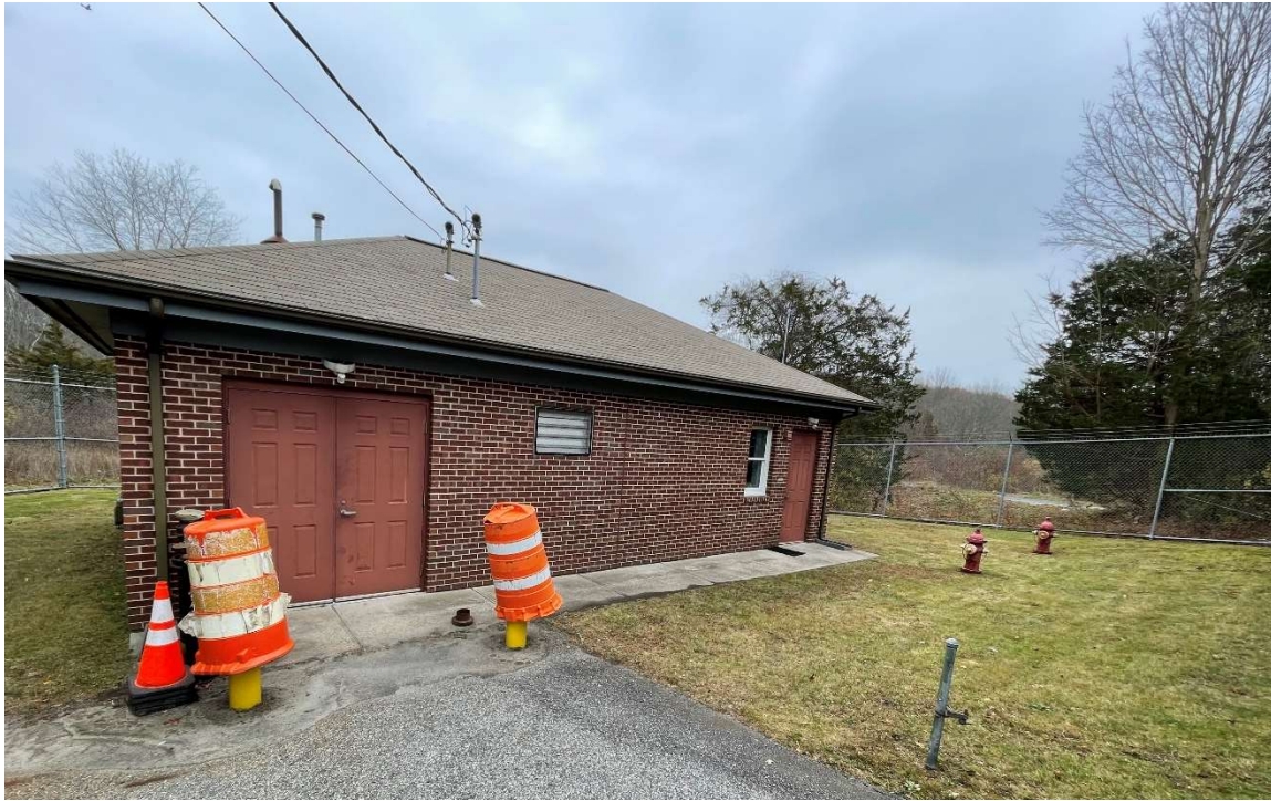
7: Limerock Pump Station Exterior
