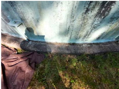
Exposed Foundation Photos
