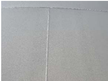
Middle East Wall Section- Photo of welds
