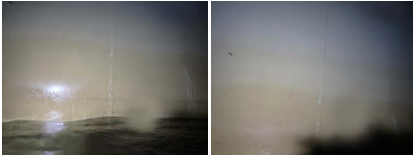
Upper North Wall Section- Photo of welds
