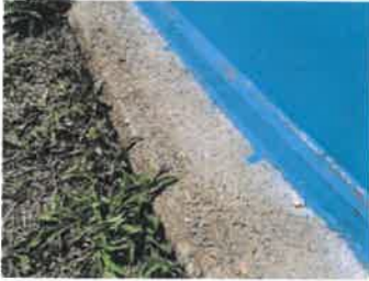
Exposed Foundation Photos
