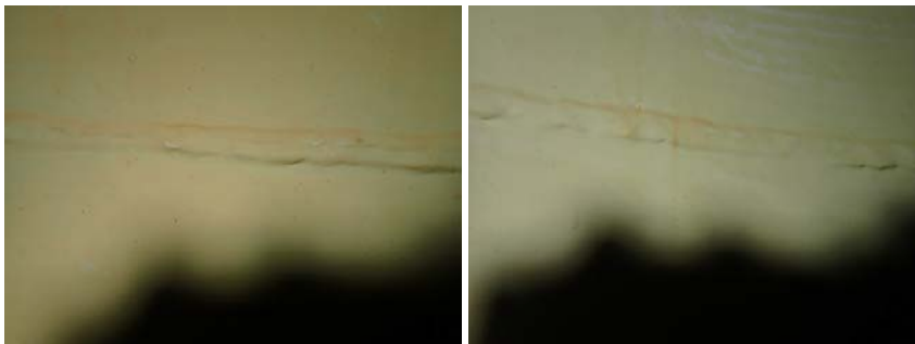
Lower East Wall Section- Photo of welds
