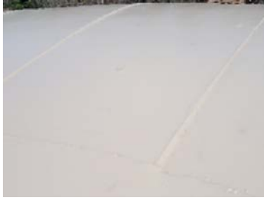
South Quadrant- Photo of welds
