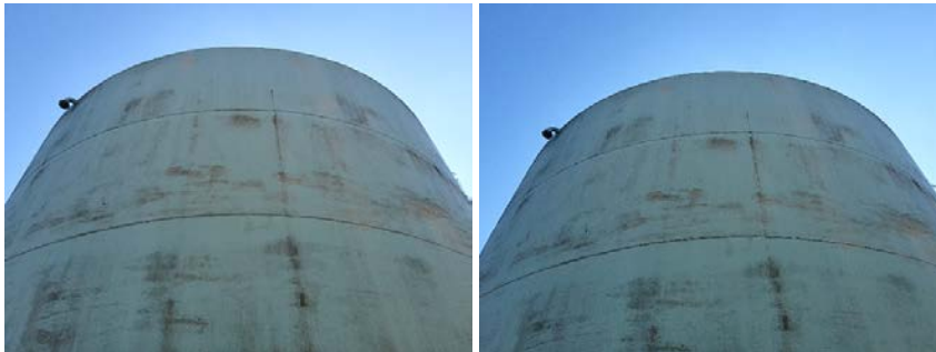
Upper West Wall Section- Photo of welds
