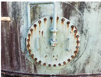
Exterior Manway 1 Photos
