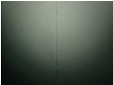
Lower East Wall Section- Photo of welds
