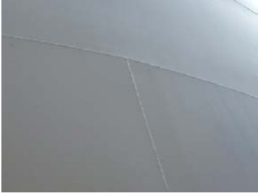
Middle North Wall Section- Photo of welds
