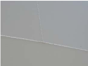
Lower North Wall Section- Photo of welds
