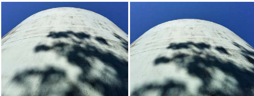
Middle East Wall Section- Photo of welds
