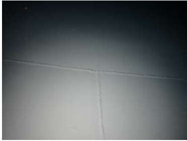
Lower North Wall Section- Photo of welds
