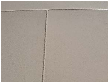
Lower South Wall Section- Photo of welds
