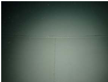
Middle East Wall Section- Photo of welds
