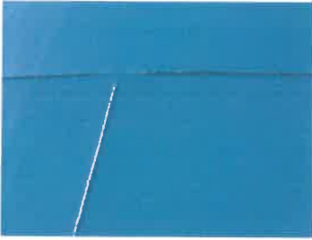
Middle North Wall Section- Photo of welds
