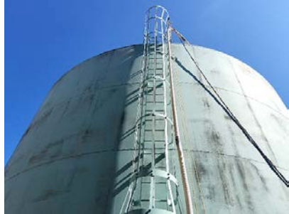
Exterior Ladder Photos
