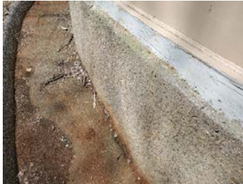
Exposed Foundation Photos
