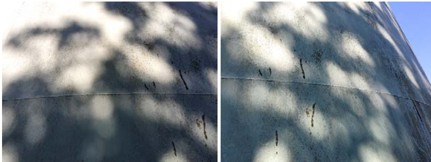
Lower East Wall Section- Photo of welds
