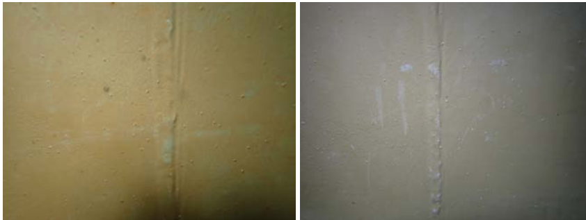
Middle South Wall Section- Photo of welds
