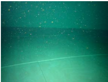
Overall Photo of Interior East Floor Quadrant
