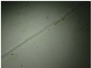
West Quadrant- Photo of welds
