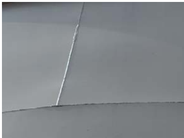
Upper East Wall Section- Photo of welds
