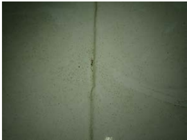
East Quadrant- Photo of welds
