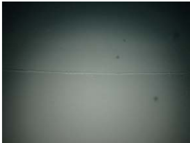
Upper South Wall Section- Photo of welds
