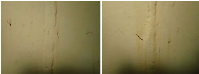
Lower North Wall Section- Photo of welds
