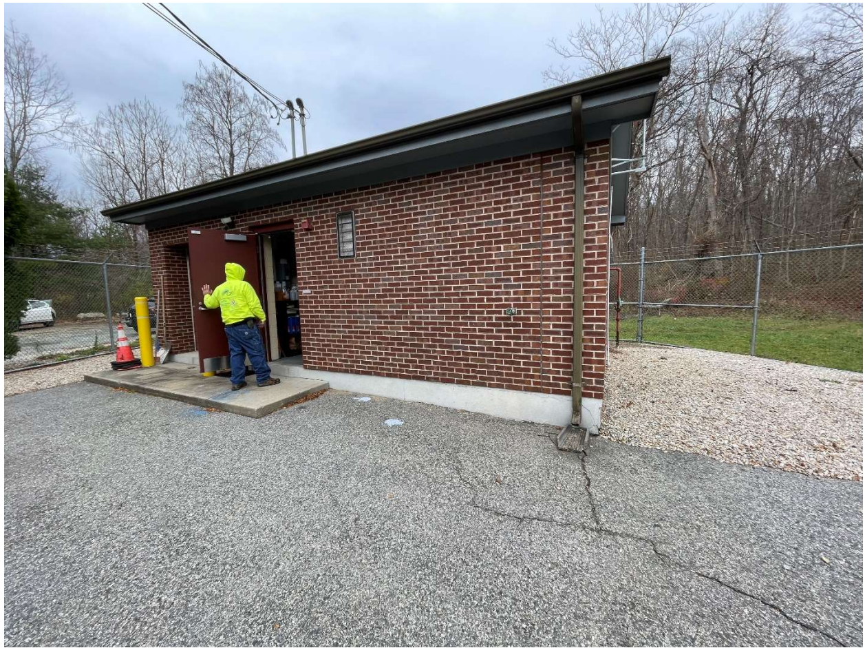
9: Davis Pump Station (Log Road Pump Station) Exterior
