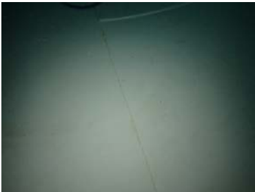
North Floor Aesthetics Photos
