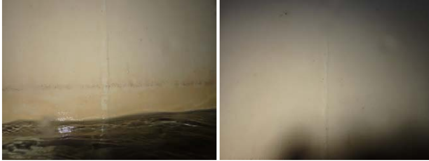
Upper South Wall Section- Photo of welds
