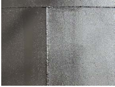
Middle South Wall Section- Photo of welds
