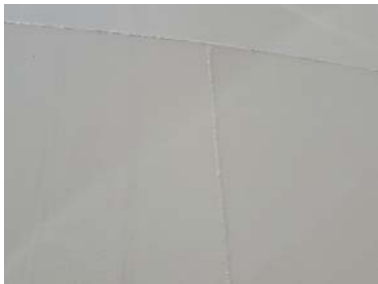
Lower East Wall Section- Photo of welds
