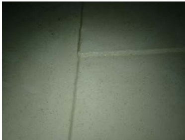
South Quadrant- Photo of welds
