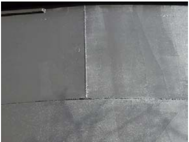
Upper South Wall Section- Photo of welds
