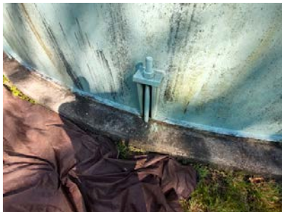
Anchor Bolts Photos
