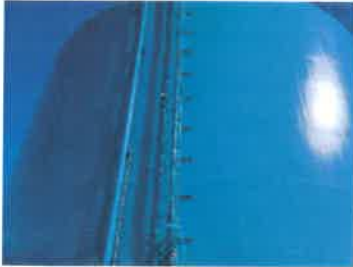
Exterior Ladder Photos
