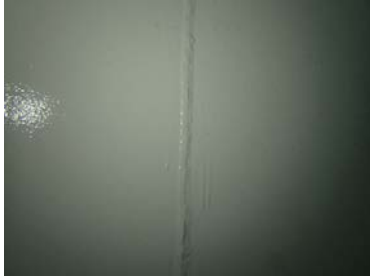
Lower South Wall Section- Photo of welds
