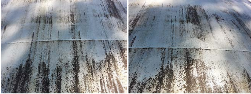
Lower South Wall Section- Photo of welds
