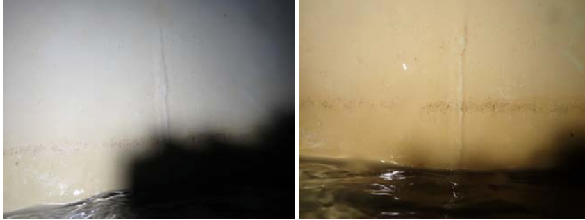
Upper West Wall Section- Photo of welds
