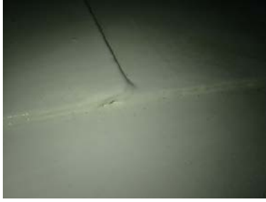
North Quadrant- Photo of welds
