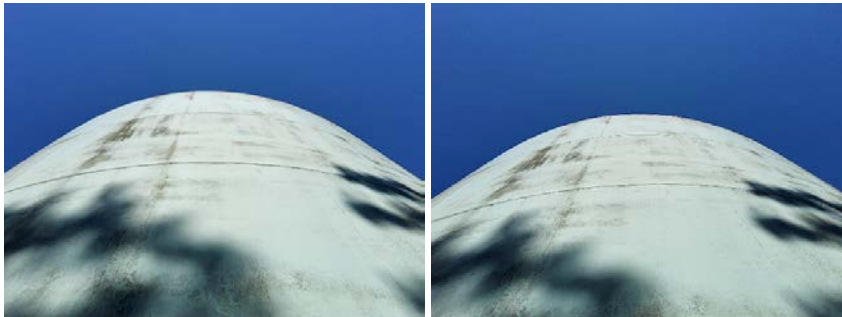
Upper East Wall Section- Photo of welds
