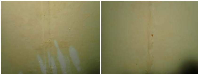
Lower South Wall Section- Photo of welds
