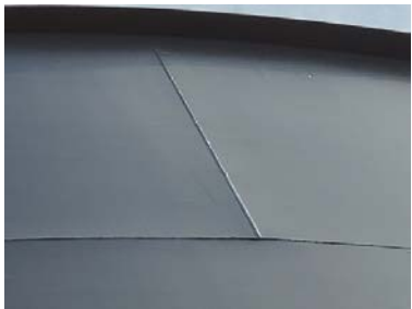
Upper West Wall Section- Photo of welds
