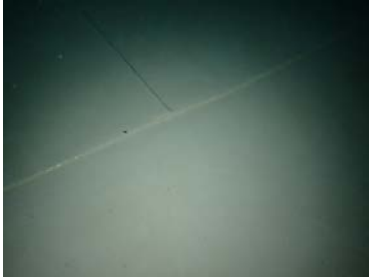
After Sediment Removal
