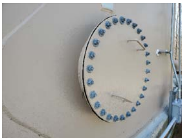
Exterior Manway 1 Photos
