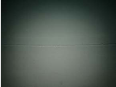
Lower West Wall Section- Photo of welds
