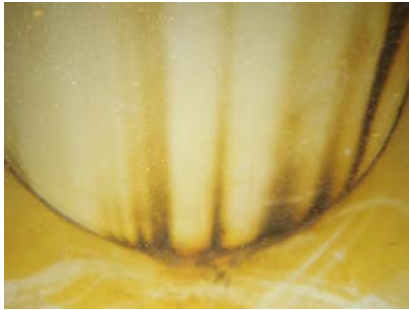
Interior Manway Photos
