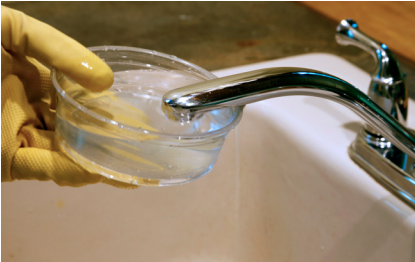
Soaking the tap with the bleach solution
