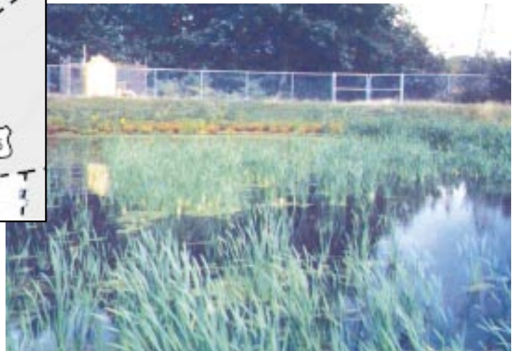
Constructed wetland in the Abbott Run watershed treats stormwater runoff. Photo courtesy RI NRCS
